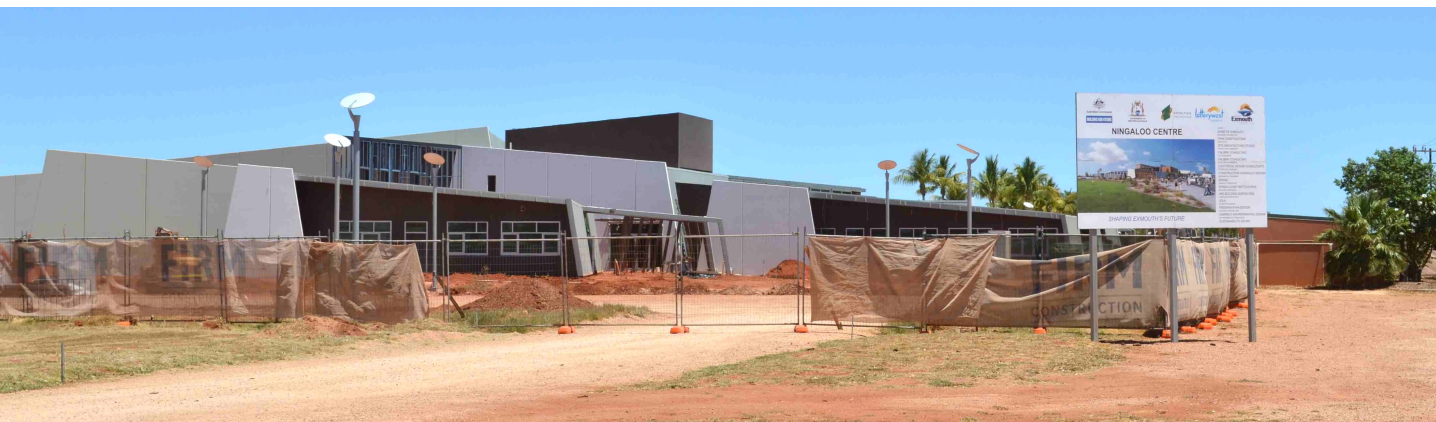
Above: Construction of Ningaloo Centre
