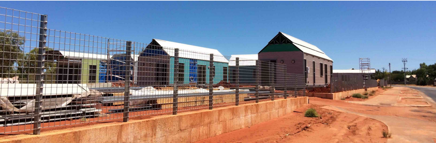
Below: Construction of Lefroy Street Affordable Housing Development
